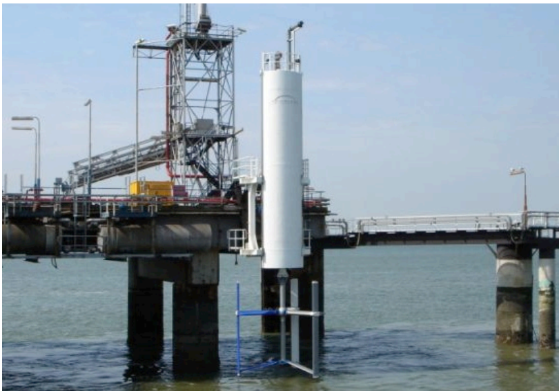
Figure 8 C-Energy project in the Westerschelde (2009), a 30kWp grid-connected vertical axis tidal turbine at a jetty of Zeeland Refineries near Borselle.
